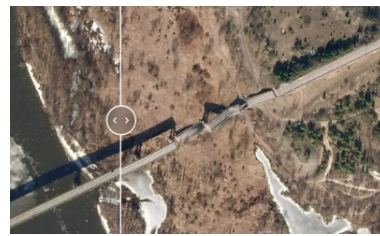
(b) Destroyed road at Kamaryn-Slavutych.
